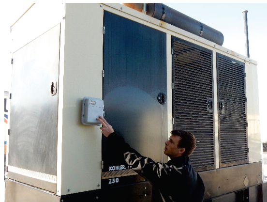
Figure 2 ADRES NEMA Case Recommended Installation Location.
