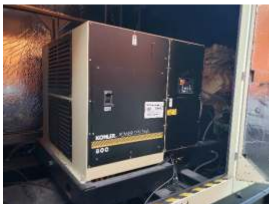
Figure 2 Open the double doors to access the DEC3000 controller.
