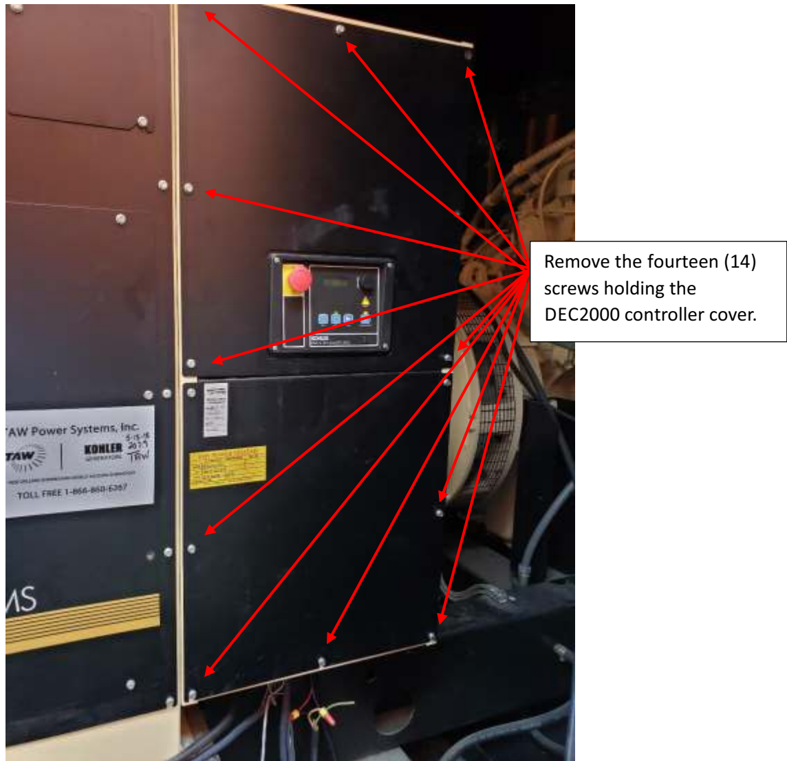
Figure 3 DEC3000 Control Enclosure Screws.
