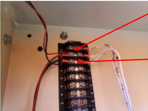
Figure 11 ADRES and Modbus Splitter Module Power Supply Terminal Board.
