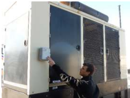
Figure 2 ADRES NEMA Case Recommended Installation Location.
