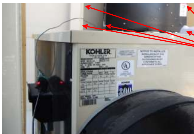
Figure 2 Control Enclosure Lid Removal
