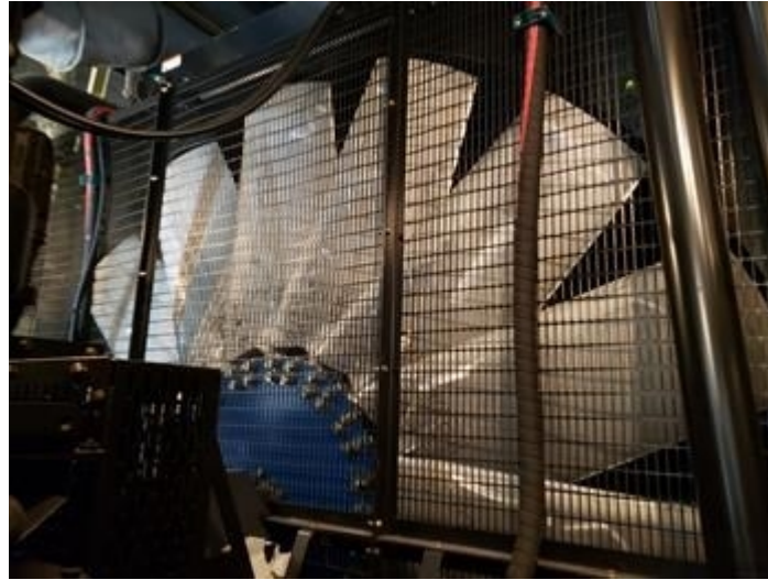
Radiator Fan After Cleaning
